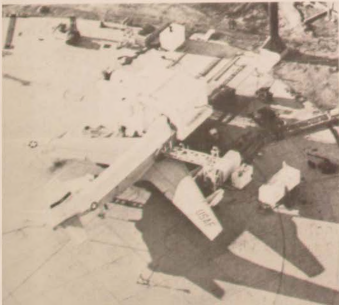
In 1981 the Air Force began field testing of the Airborne Laser Laboratory (ALL), shown above in flight. This highly modified NKC-135 aircraft is the test bed for the Air Force Weapons Laboratory's laser tests in an airborne environment. . . . The fuel farm (upper right, below) has storage tanks for laser fuels. The ALL is connected to the laser fuels servicing station, which is forward of the right wing and connected to the fuselage over it.
